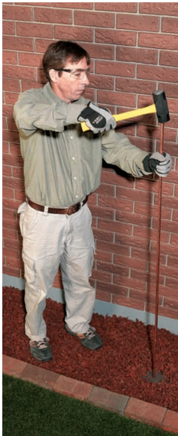
A pair of 8-ft.-long metal grounding rods are driven into the earth next to your house to provide a path to ground for your home wiring system.
