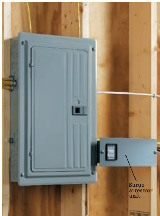
A whole-house surge arrestor is an inexpensive defense against expensive damage from high-voltage shocks caused by lightning strikes and power surges. Most models install next to the main panel.
