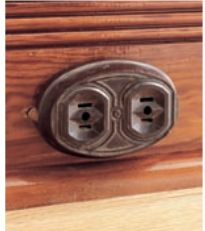
Surface-mounted receptacles were popular in the 1940s and 1950s for their ease of installation. Wiring ran behind hollowed-out base moldings. These receptacles are usually ungrounded.
