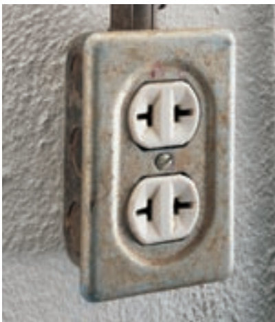
Ceramic duplex receptacles were manufactured in the 1930s. They are polarized but ungrounded, and they are wired for 120 volts.
