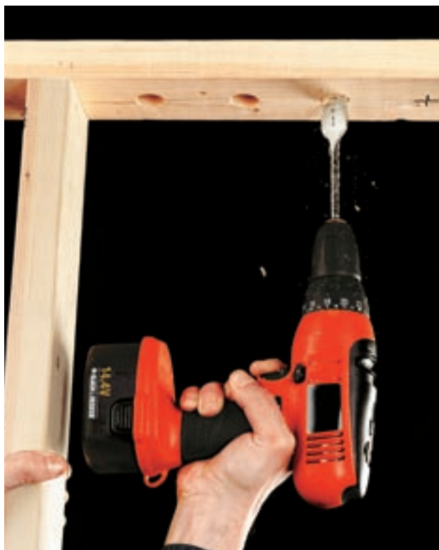
Drill 1" holes through the top plate above the distribution center. Drill holes in floor joists for running cable along the underside of house levels and from the service entrance to the distribution center.
