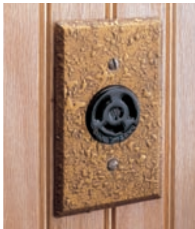
Twist-lock receptacles are designed to be used with plugs that are inserted and rotated. A small tab on the end of one of the prongs prevents the plug from being pulled from the receptacle.
