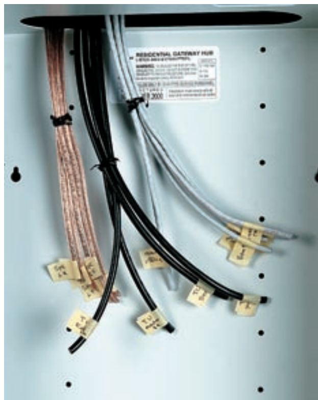
Label each run of cable and wire at the distribution center with the room and location within the room. All cables should hang even with the bottom of the distribution center.
