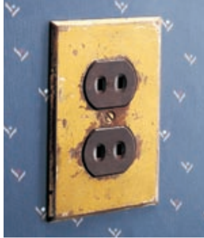
Unpolarized receptacles have same-length slots. Modern plugs may not fit these receptacles. Never modify the prongs of a polarized plug to fit the slots of an unpolarized receptacle.
