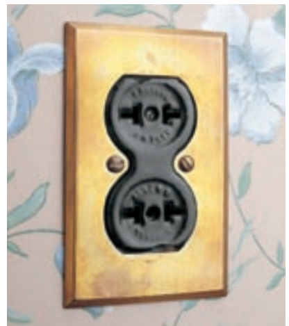
This ceramic duplex receptacle has a unique hourglass shape. It is rated for 250 volts but only 5 amps and would not be allowed by today's electrical codes.
