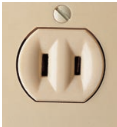
15 amps, 120 volts. Polarized two-slot receptacle is common in homes built before 1960. Slots are different sizes to accept polarized plugs.
